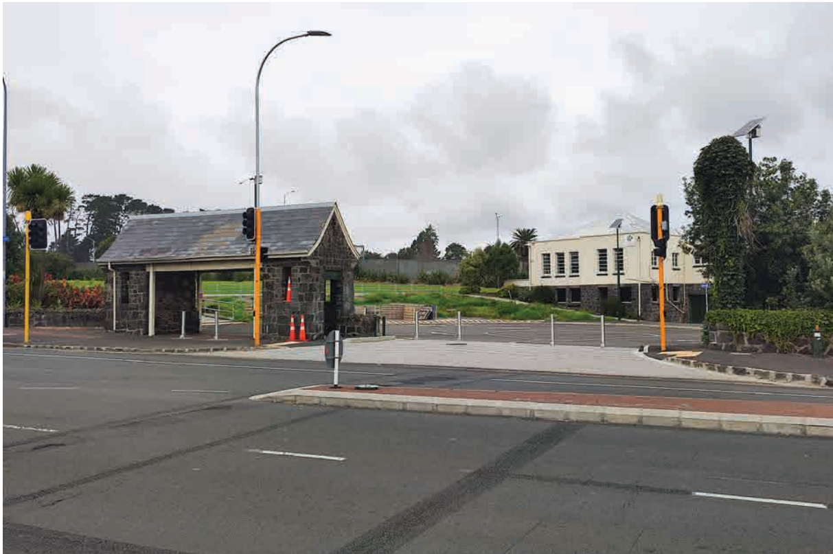
Figure 3. View of the stone arch with the clubhouse behind it.
